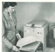
Next, the image is transferred from the plate to the offset paper master. Then it is removed and is ready for fusing.
