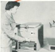
Plate is charged in Copier, then placed in Camera. The image of material to be copied is transferred directly to charged plate.
